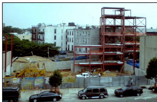
View of Universal Church project from Fulton Street, jobsite Nov. 11, 2007.
